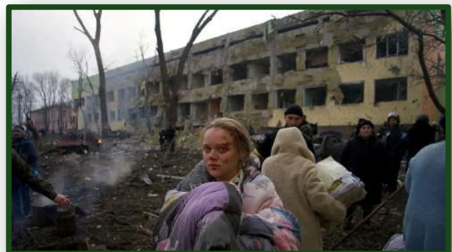
A maternity hospital that was damaged by shelling in Mariupol on Mar. 9; the Ukraine war has changed global geopolitical considerations. © AP
